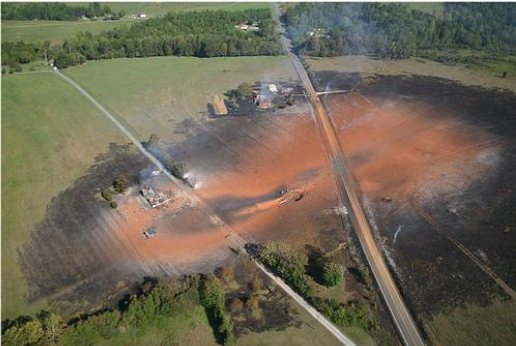
Impact area from Appomattox pipeline failure
